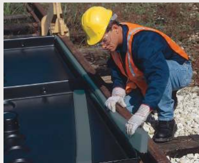
Closed-cell, polyethylene gaskets are installed to provide a seal between the Pans and rails. (Gaskets are provided.)
