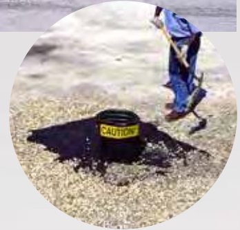
Large, 4' x 6' size is installed by placing on top of grate and securing with gravel or other aggregate.
