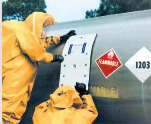
These simple devices expand a chemical resistant, flexible bladder to quickly stop potentially dangerous and costly spills.
