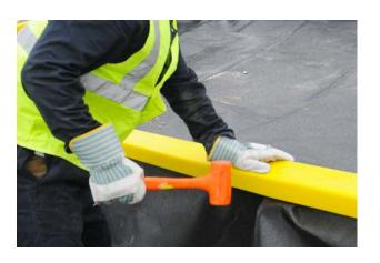
8. Place clips (two per wall / one per corner) over liner to secure it in place. (NOTE: The clips are designed to fit snugly and may require a fair amount of force to install. A rubber mallet can be helpful).
