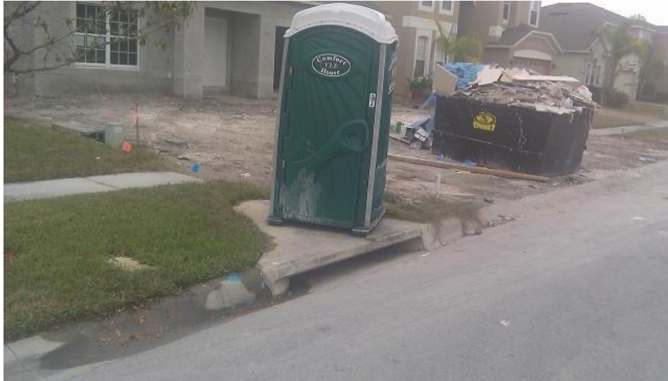
Figure 2: Absence of inlet protection on residential construction
