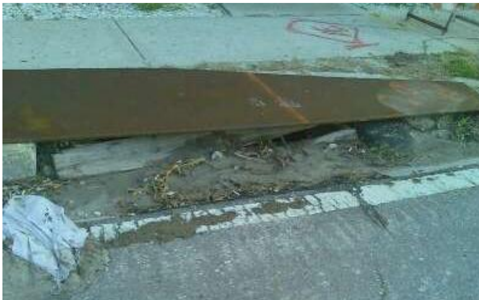
Figure 1: Lack of inlet protection
