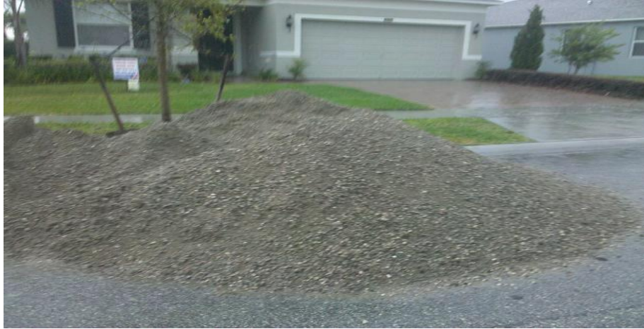
Figure 5: Improper aggregate storage
