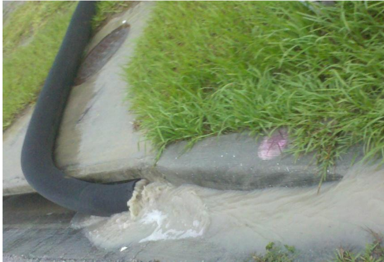
Figure 4: Improper curb inlet protection practice
