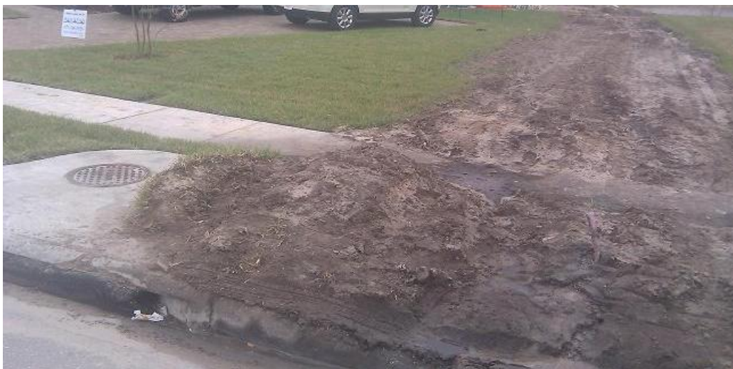
Figure 6: No source control adjacent to inlet
