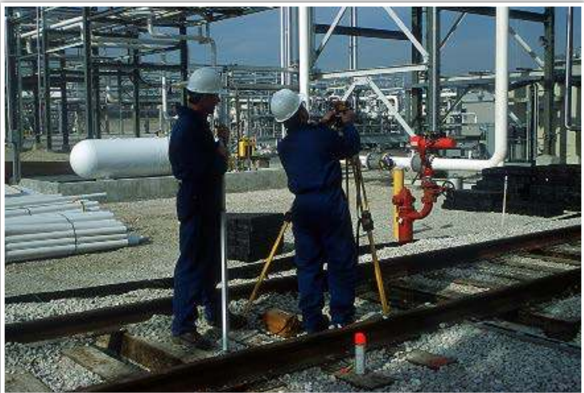
Survey to design correct slope for piping
