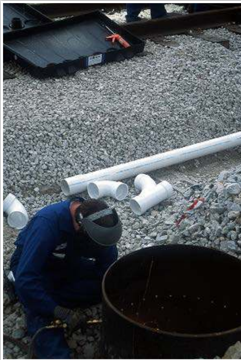
Connect pipes to sump
