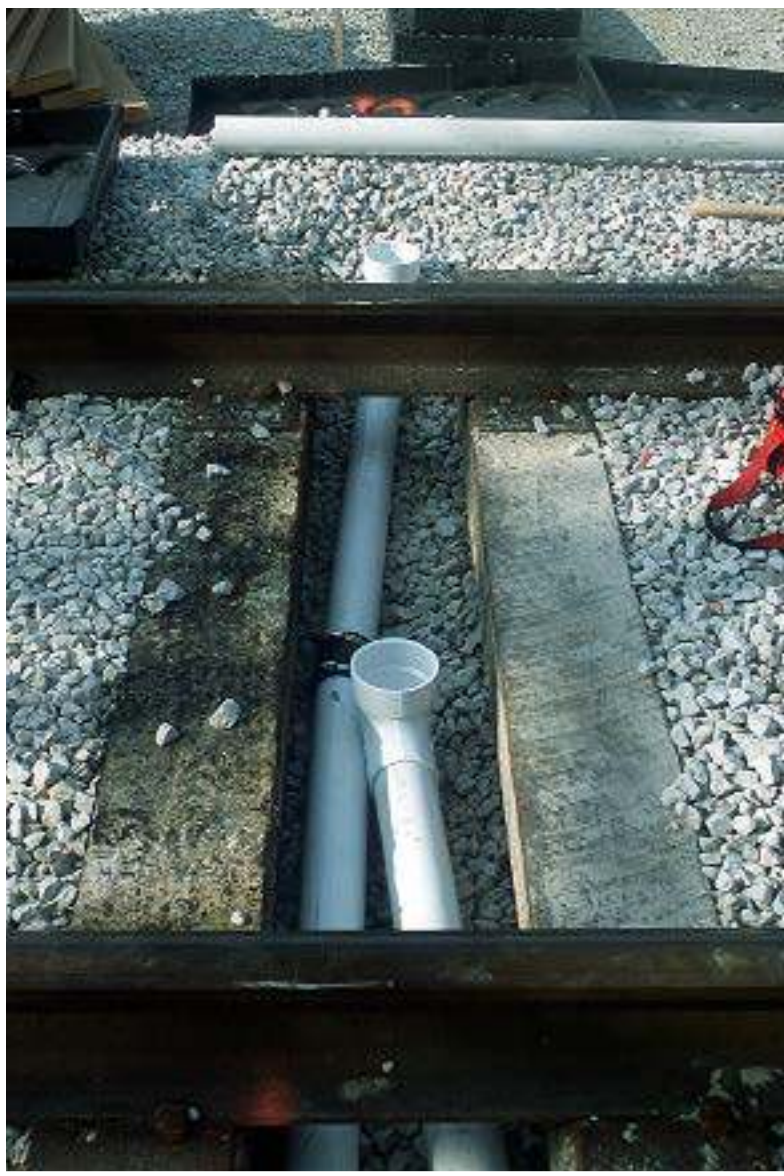
Early stage pipe installation
