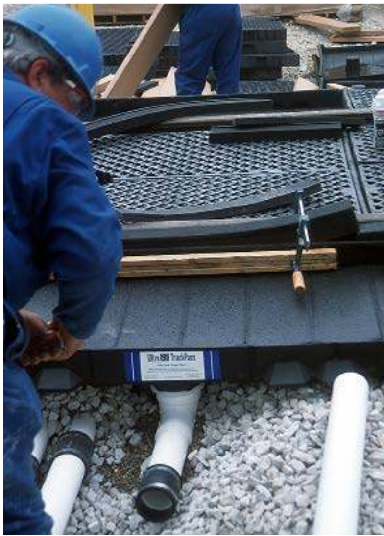
Connect pipes to Pans
