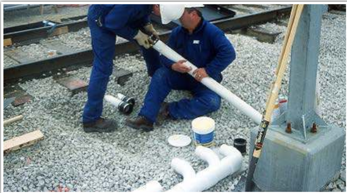
Connect pipes to Pans
