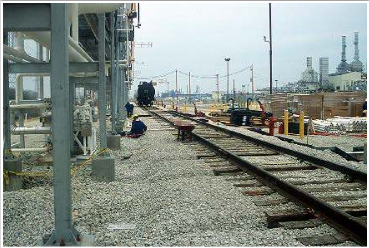
Facility siding prior to installation
