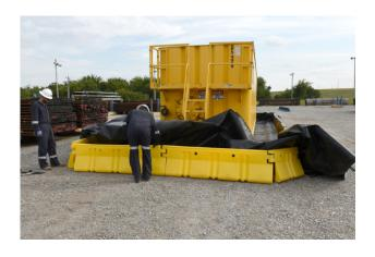
10. Once truck and/or any other equipment that will not be contained is removed, replace any walls/corners that were removed in step 6.
