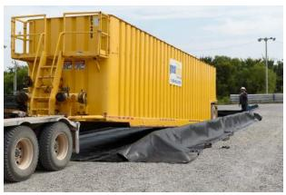
9. Carefully drive/roll container (frac tank, etc) into Containment Wall system.
