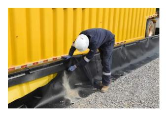
12. OPTIONAL: If desired, any excess liner material can be trimmed using a sharp utility knife.
