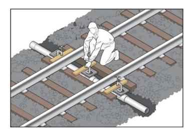
3. Backfill the void with "crush and run" sand. If possible, have additional personnel stand on the boards as added support to prevent the manifolds from moving. Pour sand around the manifold until it is just below the top of the tie. It should very gently be tapped into place to make sure it settles nicely under and around the manifold. Avoid getting sand into the drain.
