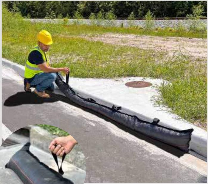
Heavy-duty, pre-installed lift loops make lifting, installing and moving quick and easy.
