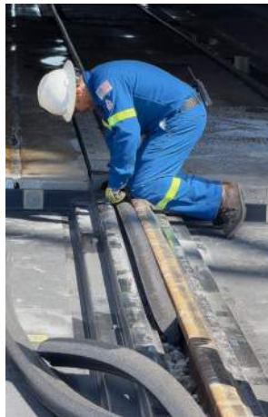
Rail Gaskets are installed between pan and rail to seal off any openings to avoid spills.
