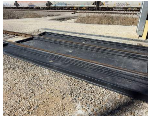
Rail Gaskets are installed between pan and rail to seal off any openings to avoid spills.
