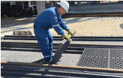
Gratings can be easily placed on or removed from pans.
