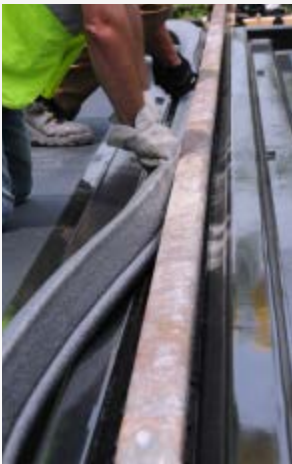
Optional rail side gaskets prevent leaking between rails and Track Pans.
