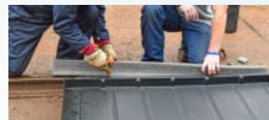
Included gaskets prevent pellets from getting between pans and rails.
